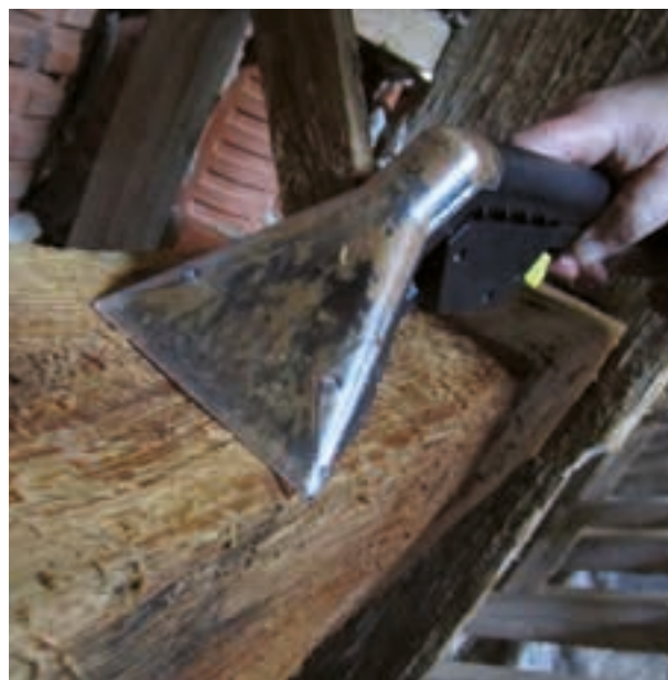
Naumburg, cathedral, testing whether the wood can be cleaned using an extraction cleaner
