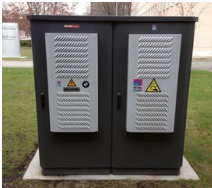
Stationary second-life battery bank for an Efficiency House Plus
