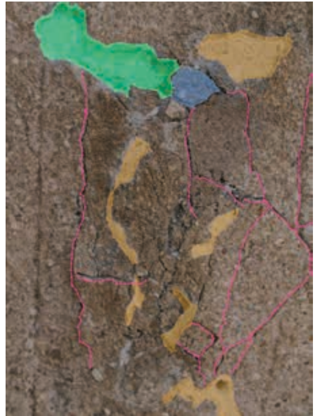
Figure 2a und 2b: Photo (a) and 3D mapping of cracks using the tracking system (b) of a hollow in the markings in the plaster in Magdeburg cathedral
