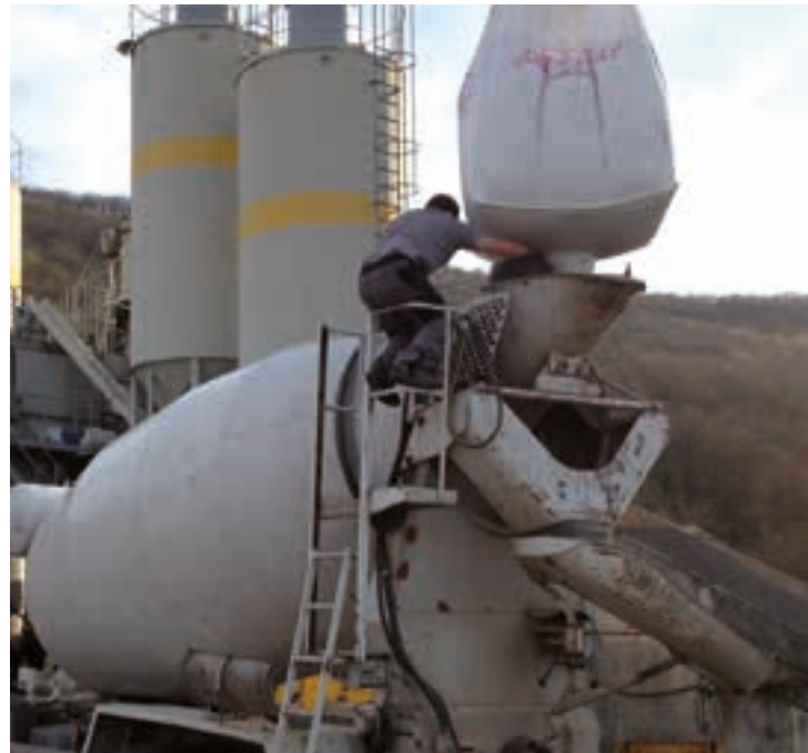
The blown glass granules being tipped from big bags into the mixer truck
