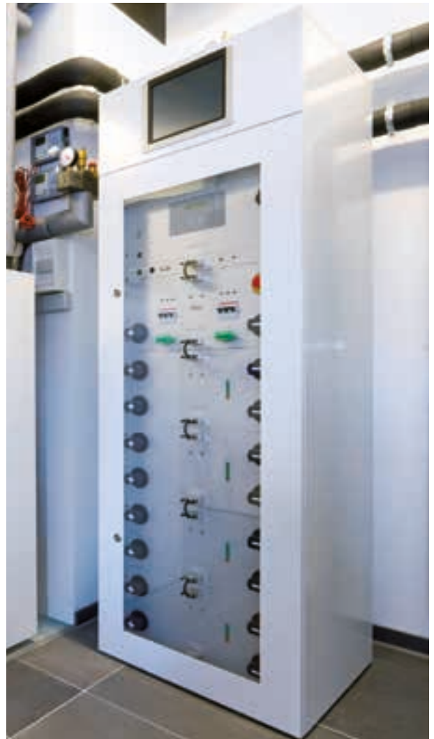
New battery storage system, capacity: 13.2 kWh
