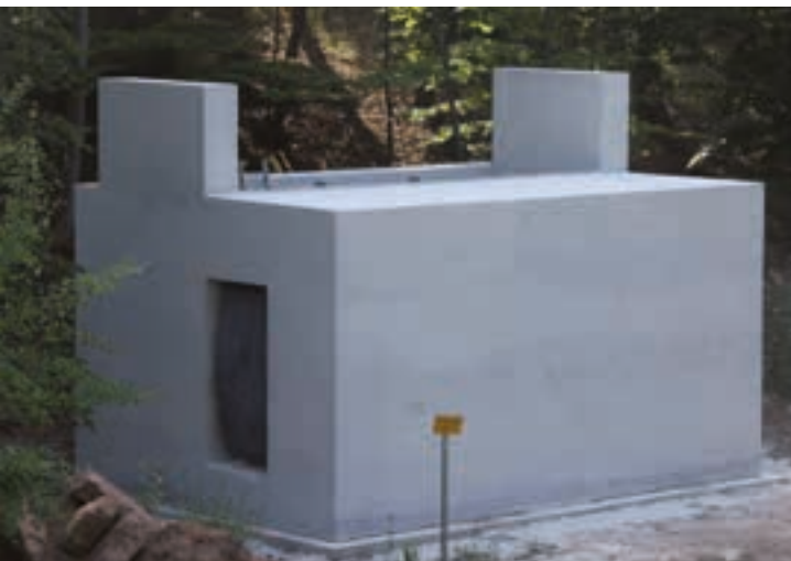
Lightweight architectural concrete building following completion of the concreting operation
