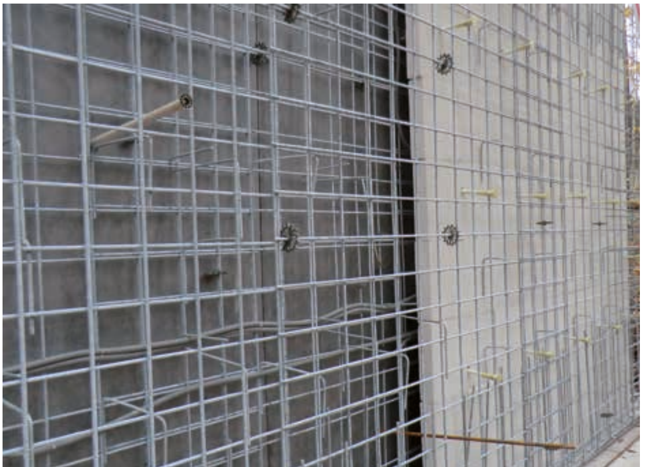
Wall of the experimental building with mineral foam core insulation
