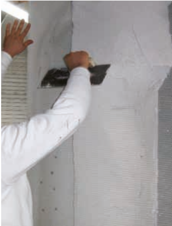
Successful plastering trials on a polystyrene model
