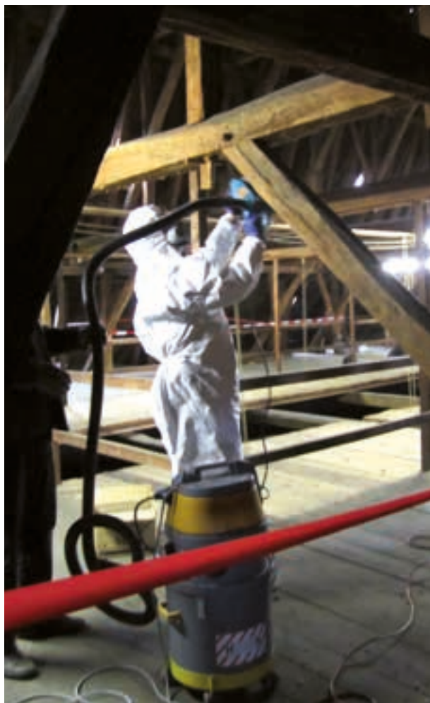
Meisenheim, Schlosskirche, testing whether the wood can be cleaned with a rotating brush
