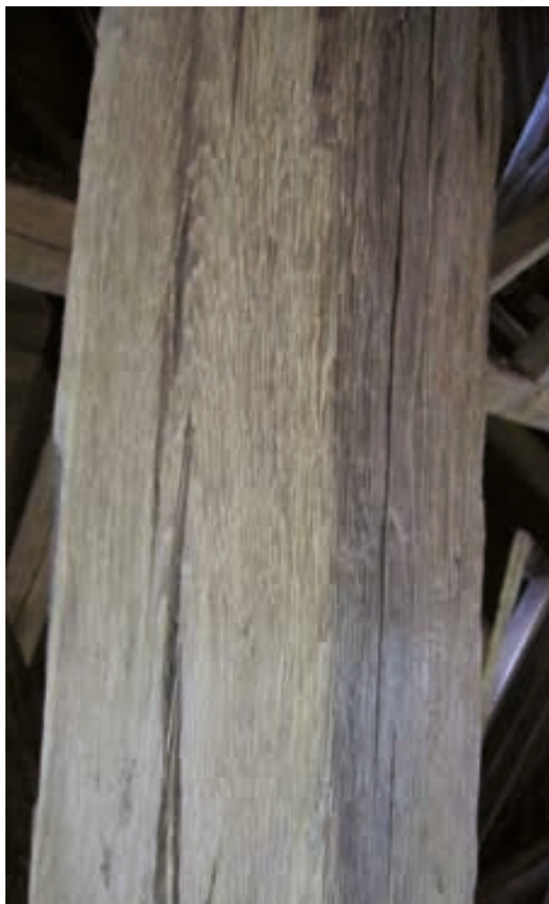
Meisenheim, Schlosskirche, surface of the oak structure after cleaning with a rotating synthetic brush
