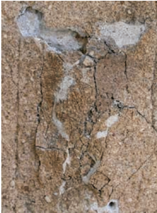
Figure 2a und 2b: Photo (a) and 3D mapping of cracks using the tracking system (b) of a hollow in the markings in the plaster in Magdeburg cathedral
